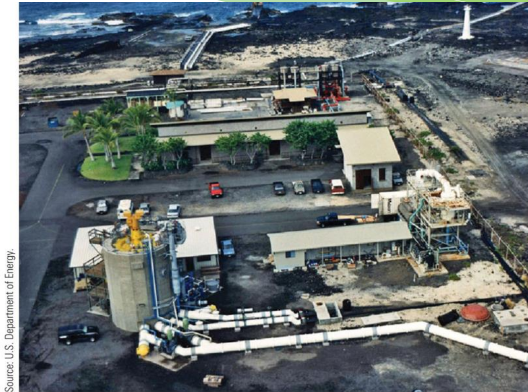
Figure 14.9: Land-based 250-kW open-cycle OTEC demonstration plant at Keahole Point, Hawaii.
